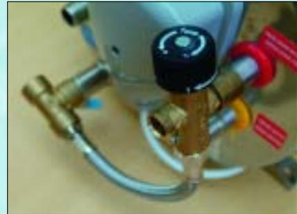
**MIXER VALVE:** The tanks from Isotemp have a mixer valve as standard. The temperature of the water to be supplied by the heater is set here. Cold water is mixed in with the hot water to attain the correct temperature.
